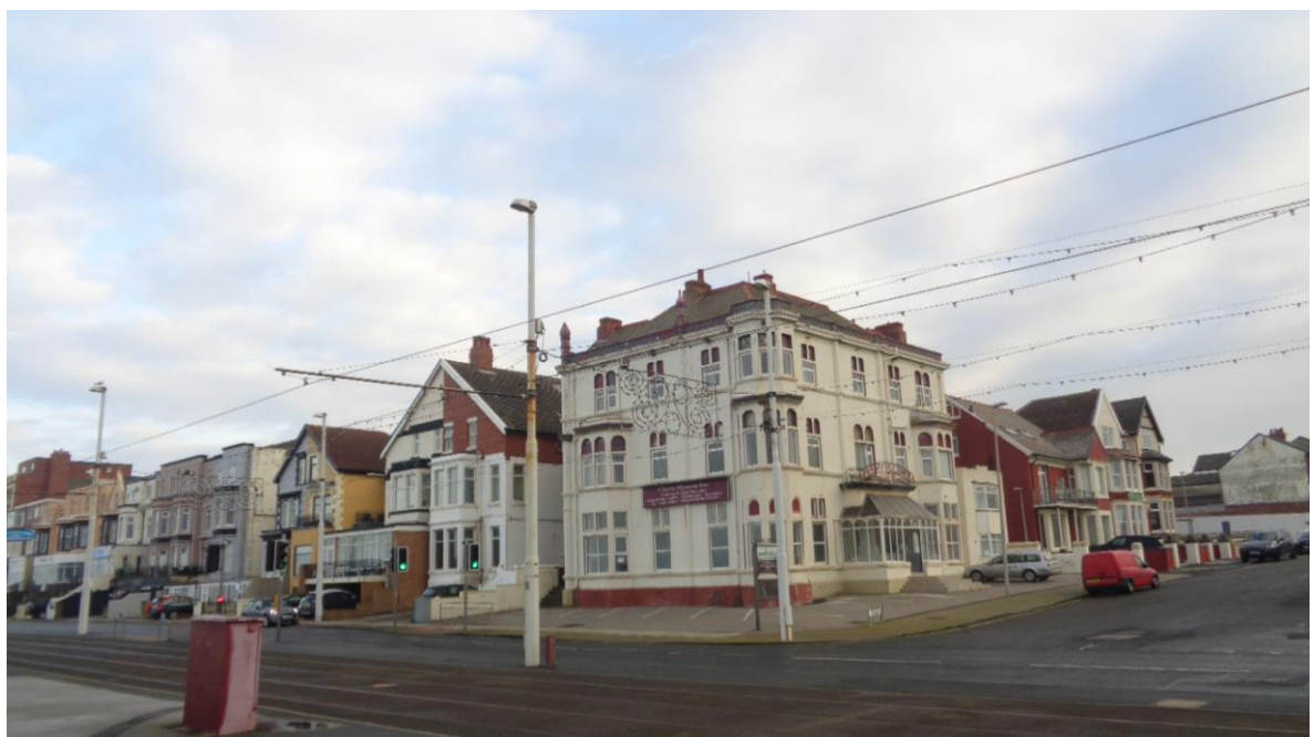
Small hotels to the north of the former Derby Baths site with a variety of sun lounges
