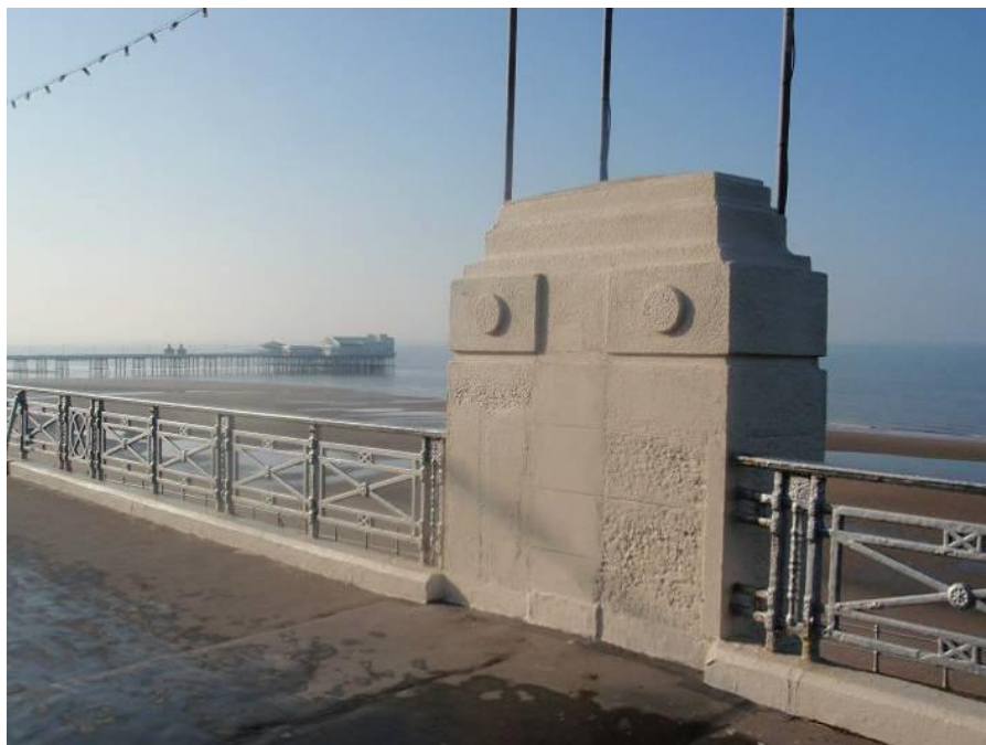
Piers and balustrades to upper walkway
