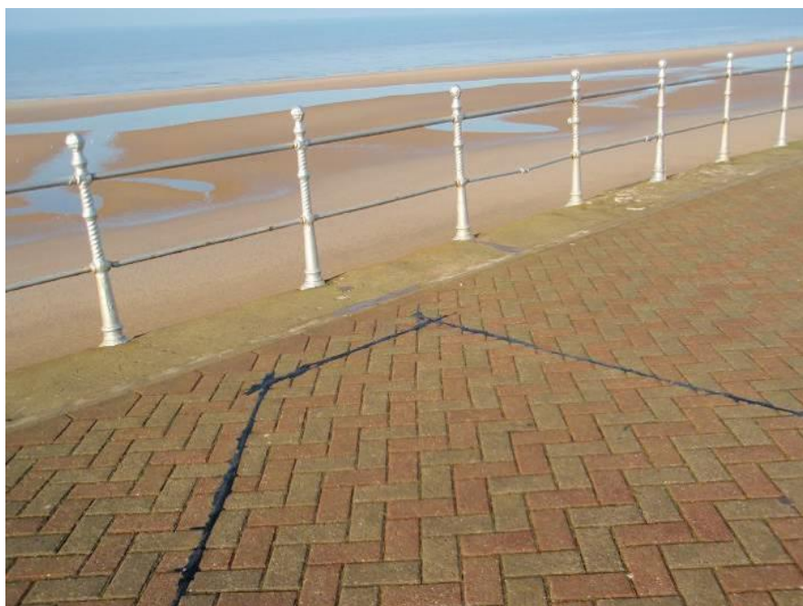
Balustrades to lower walkway
