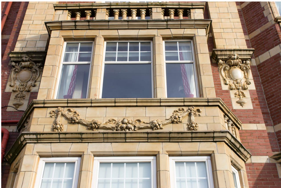
Windows with faience decoration, Cliffs Hotel
