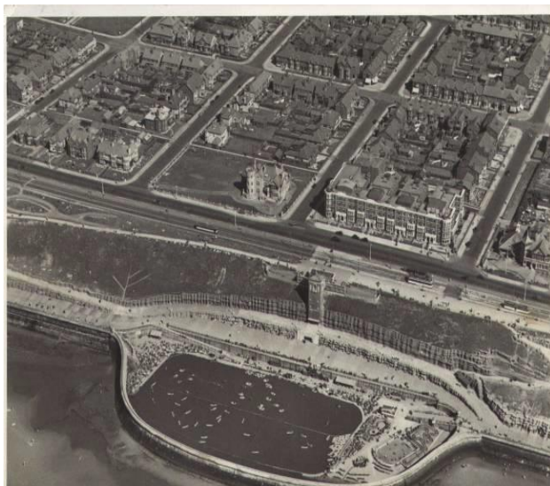
North Prom from the air, c.1930, showing part of the artificial cliffs, the cabin lift, boating pool, Uncle Tom's Cabin pub, and 'The Castle', a private residence
