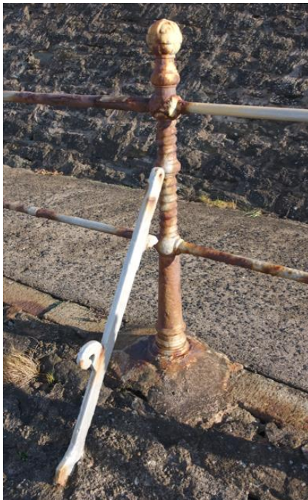
Corroding balustrade
